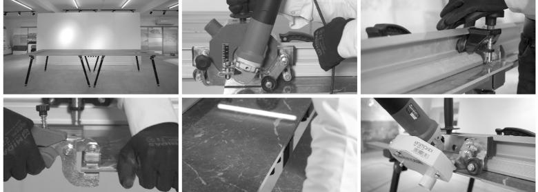
• RAK Ceramics recommends the use of special designed devices for handling as well as cutting and laying of big slabs.
