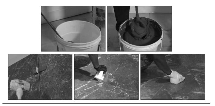
Fill the joints with a special grout float or rubber squeeze without leaving any gaps or steps. Remove any excess grout and leave
